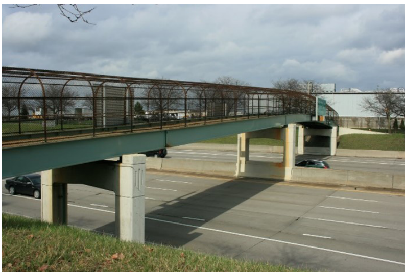
Figure 65: Pedestrian overpass across a freeway
