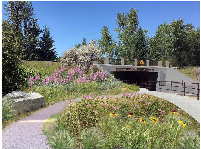
Figure 39: Pedestrian and cyclist underpass for I-90
