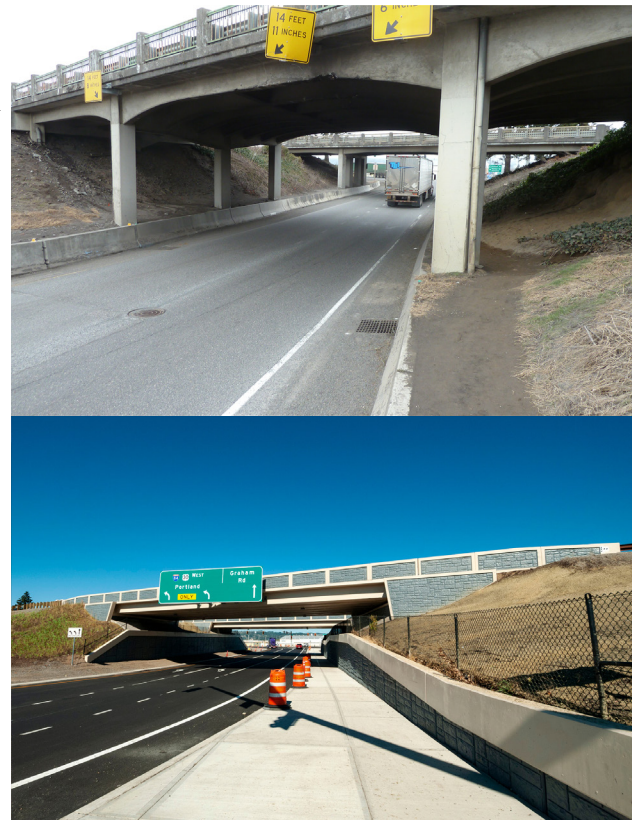
Figure 41: I-84 Graham Road Bridges, Oregon DOT
