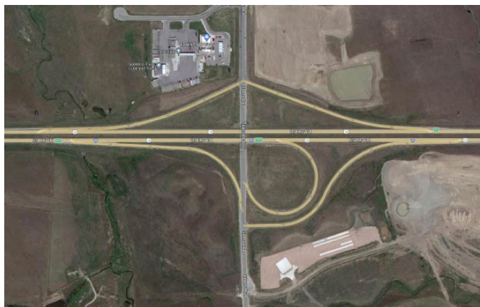
Figure 44: Exit 67 on Interstate 90 is overly complicated
